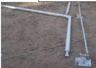
3. Assembled leg, eaves joint, roof beam
