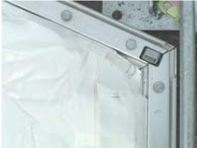
11. Roof cloth installed in the inner round slot. Illustration shows the eaves joint
