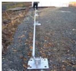
1. Ground plates installed with tension tubes.
