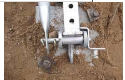
6. Corner plate Z, leg, hairpin spring, tension tube, hairpin spring, installed on foot plate with foot print
